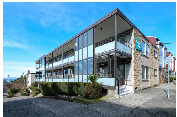
301 14th Ave E, Capitol Crest or Shermily Apartments
