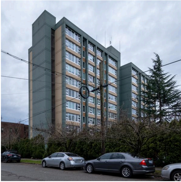
525 14th Ave E, Capitol Park Apartments
