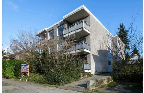
224 and 228 11th Ave E, Lurline Apartments
