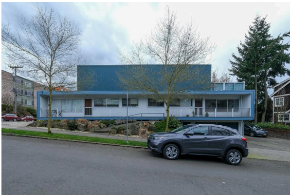
1111 E Harrison St, Harrison Modern Apartments
