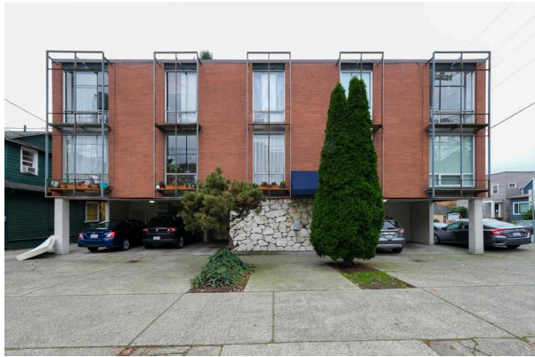
129 11th Ave E, Casa Verde Apartments
