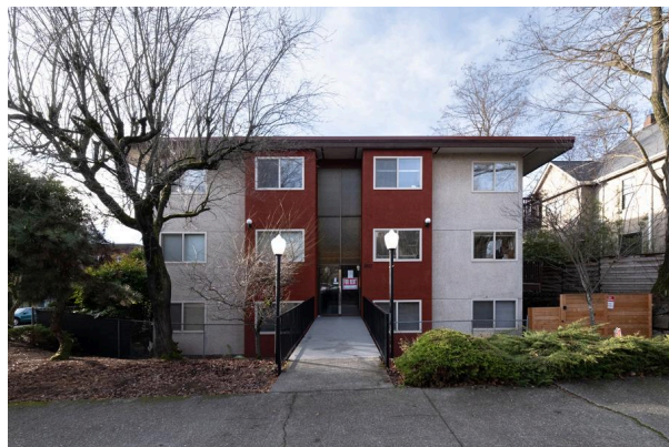
1803 14th Ave, Hollywood Apartments
