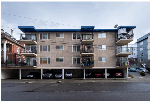
600 E Olive St, Centennial or Belcrest Apartments
